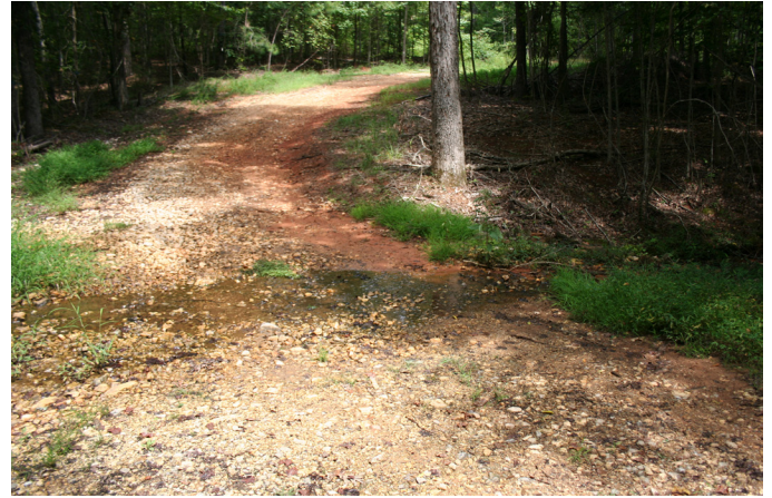
Constructed ford (Photo credit: Janice Dyer)
